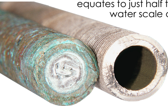
Chiller tubes before and after RYDLYME
