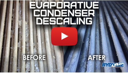
Watch as RYDLYME Descaler dissolves scale build up from this evaporative condenser!
