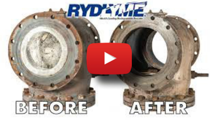
Watch as RYDLYME Descaler safely dissolves struvite from this check valve!
