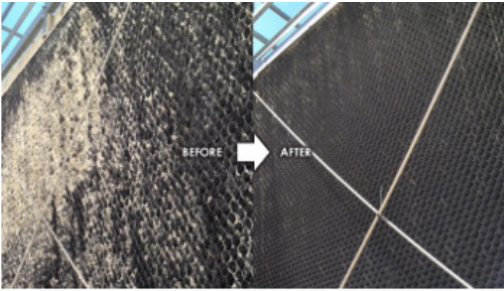
Cooling tower before & after RYDLYME chemical descaler
